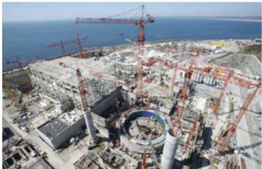
Figure 5: Flamanville 3 under construction 73 .
